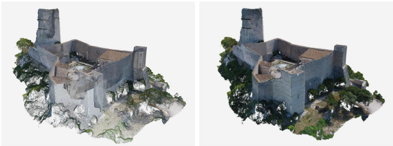
Fig. 1. Digital representation of Rocca Janula, in the current state with the gaps (left, photogrammetric survey processing by drone) and in the possible post-intervention condition of insertion of 3d printed material (right, textured model).
