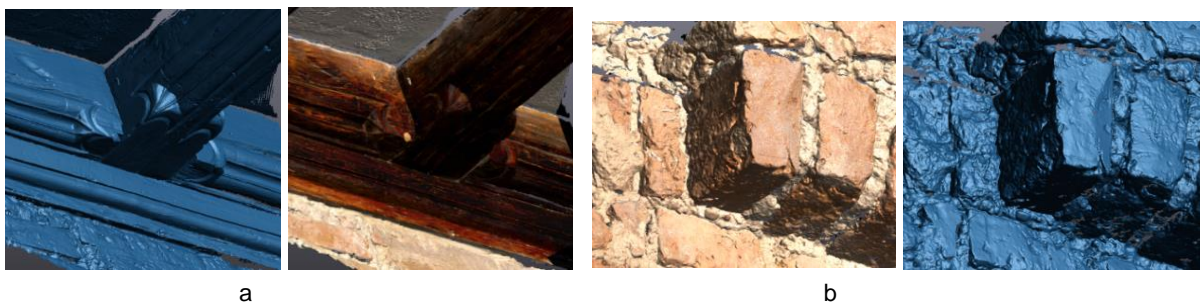
Fig. 2. 3D examination of the detail with complex geometry; 2a. Examination of wooden beams, 2b, examination of brick structure.
