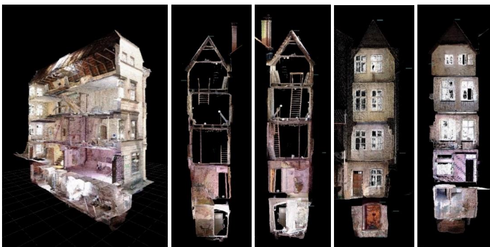
Fig. 1. 3D laser scanning of the tenement house, Poznań, Poland
