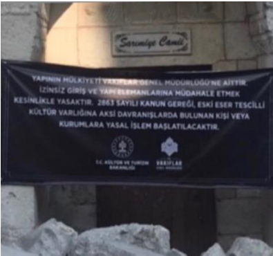
Figure 5- Damaged cultural property sign (Architect Birsen Parlar archive)
