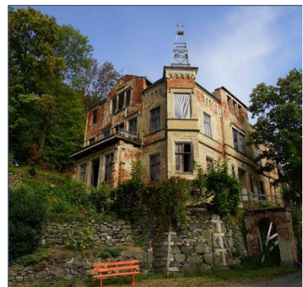
demonstration object at Liebau, Saxonia, Germany.
